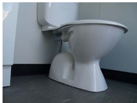
Inside : Concealed Plumbing and Electrical Cabling
